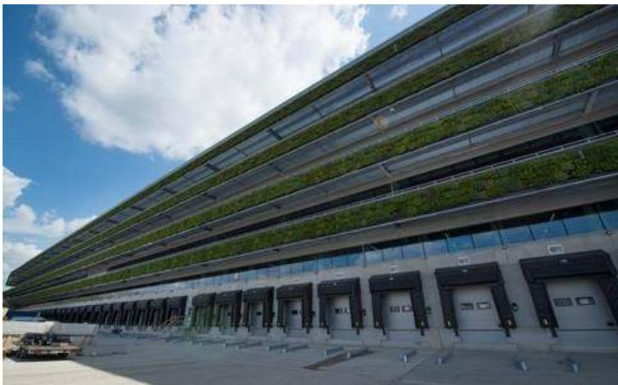
This building uses Mobilane<sup>®</sup> Green screen, which is a pre-grown pre-cultivated screen that can provide disguising and also a security perimeter.
